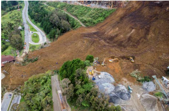
Figure 13- Landslide at Medellín-Bogotá highway in 2016 (Source: eNCA)
